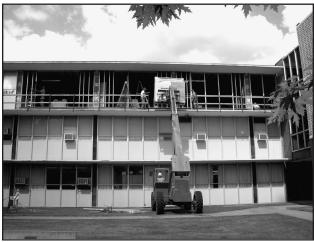
Workers prepare to install new energy-efficient windows and walls on the south side of the middle wing. Yes, it was completely open.
